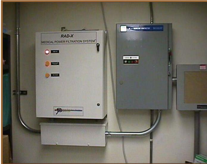
Rad-X Filter installed for CT System
